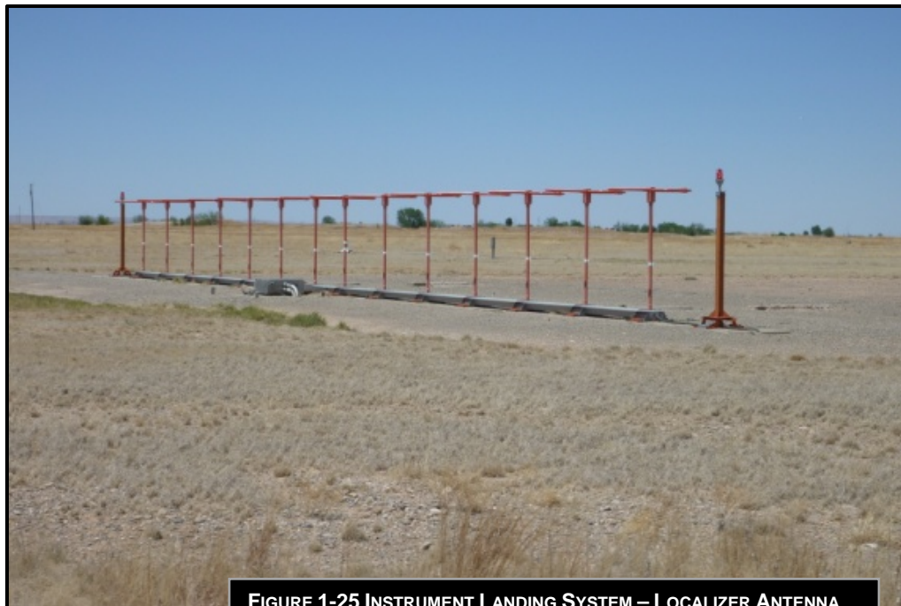
FIGURE 1-25 INSTRUMENT LANDING SYSTEM – LOCALIZER ANTENNA
