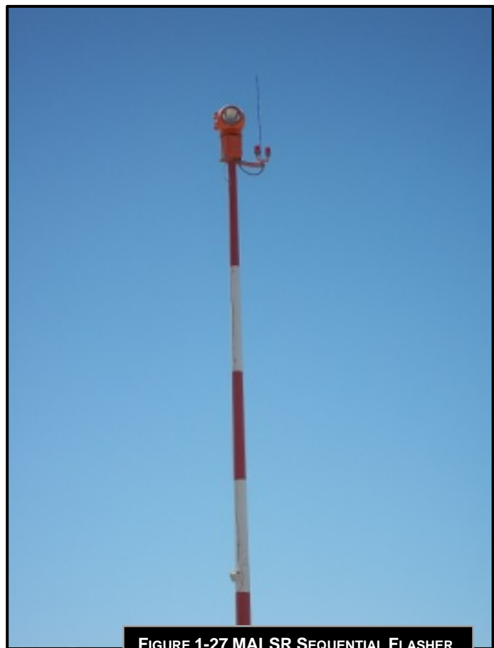
FIGURE 1-27 MALSR SEQUENTIAL FLASHER
